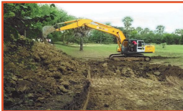
Pond excavated by heavy machinery
