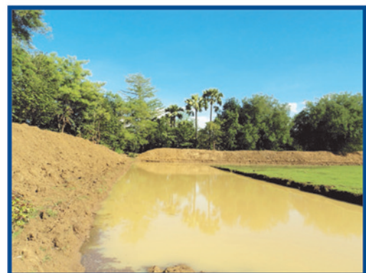
Pond harvested rain water after digging
